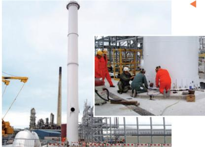
The LIEBIG **ULTRAPLUS** undercut anchor can resist high loads problem-free, even at close anchor spacings. The application shown required a load capacity of 294 kN per anchor.
