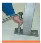
Apply the specified installation torque using a calibrated torque wrench - the ULTRA-PLUS undercut anchor is now installed and can resist loads immediately!
